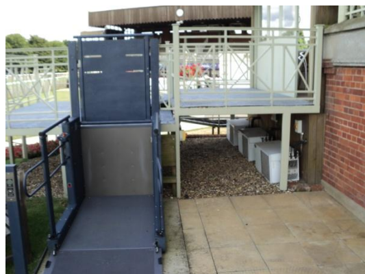
Accessible lift to viewing platform next to integrity tower
