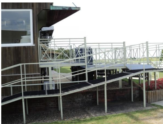
Viewing platform next to integrity tower
