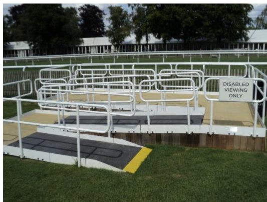
Viewing platform in Premier Enclosure Racecourse side
