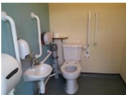
Accessible toilet Grandstand and Paddock Enclosure
