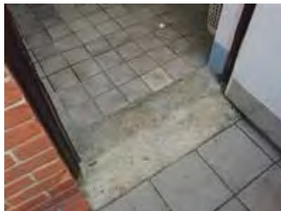
Level change in Courtyard Disabled toilet.
