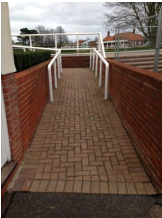
Access ramp to the Frankel Lounge
